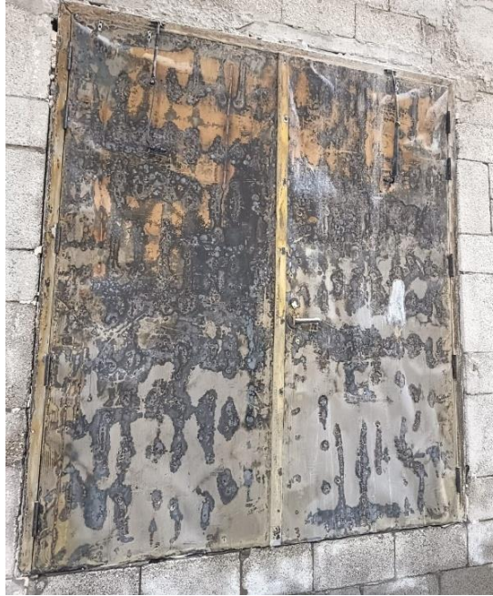
Figure 12: The exposed face after the test.
